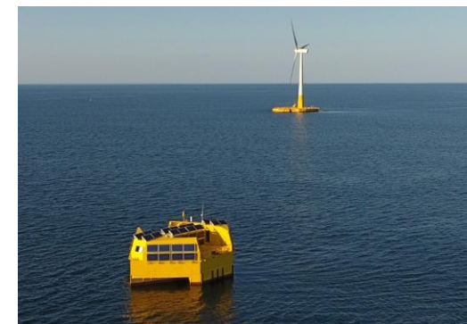
Offshore hydrogen production facility 3
