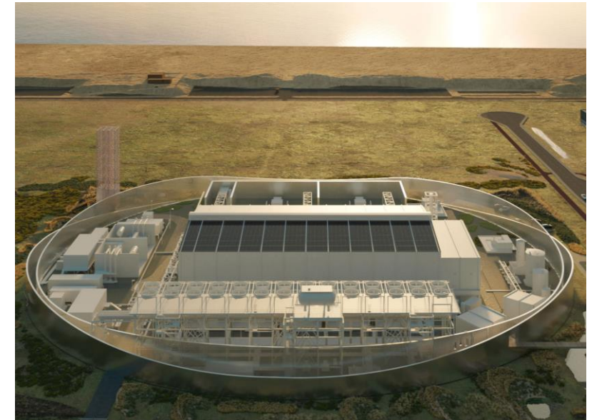
Project Holland Hydrogen I, a 200MW Electrolyser planned to be constructed in the Port of Rotterdam 4
