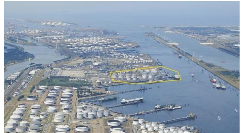
OCI's ammonia import terminal in Port of Rotterdam (bordered by yellow line) 2
