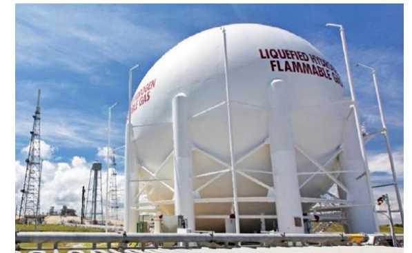
LH 2 storage at NASA (source: NASA)
