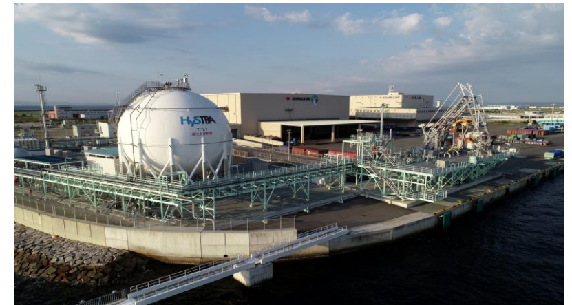
Liquefied Hydrogen Receiving Terminal in Japan 3
